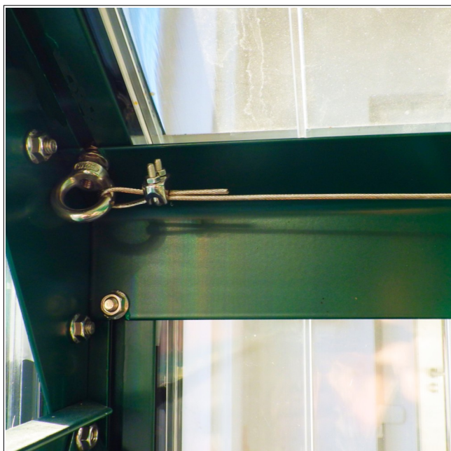
Abb. 1 (C. Drahtseil an Öse fixieren)
